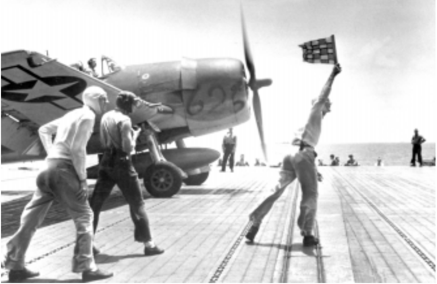
Hellicat pilot about to get the signal to take off. Note drop tank and flaps in full “down” position. (Corbis)
